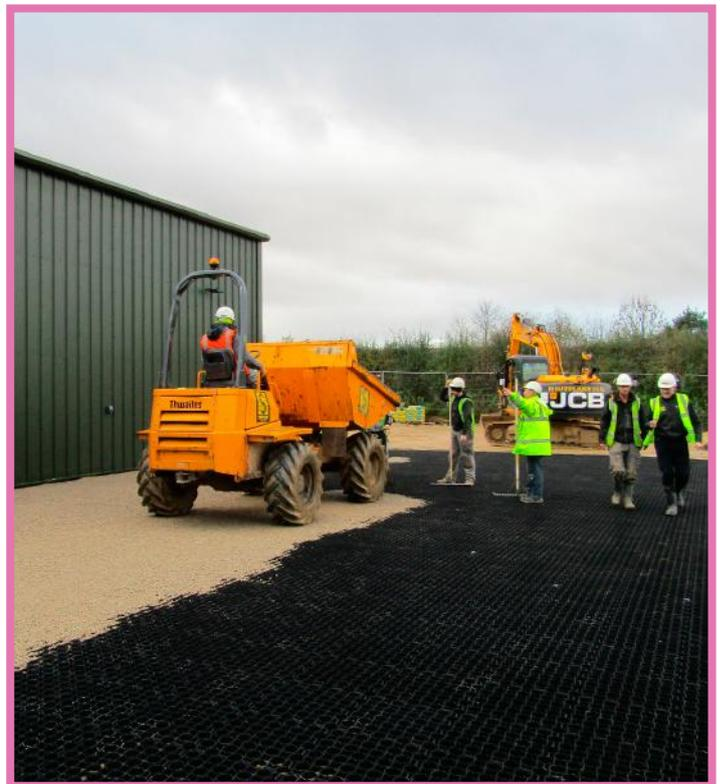
1. Mark out and excavate area to required depth, sub-base depths required vary dependent on traffic load being applied. Table 1 indicates sub-base depths required. Remember to add the depth of the GRB PLUS to the figures in the table if the GRB PLUS is to finish flush to the surface.
